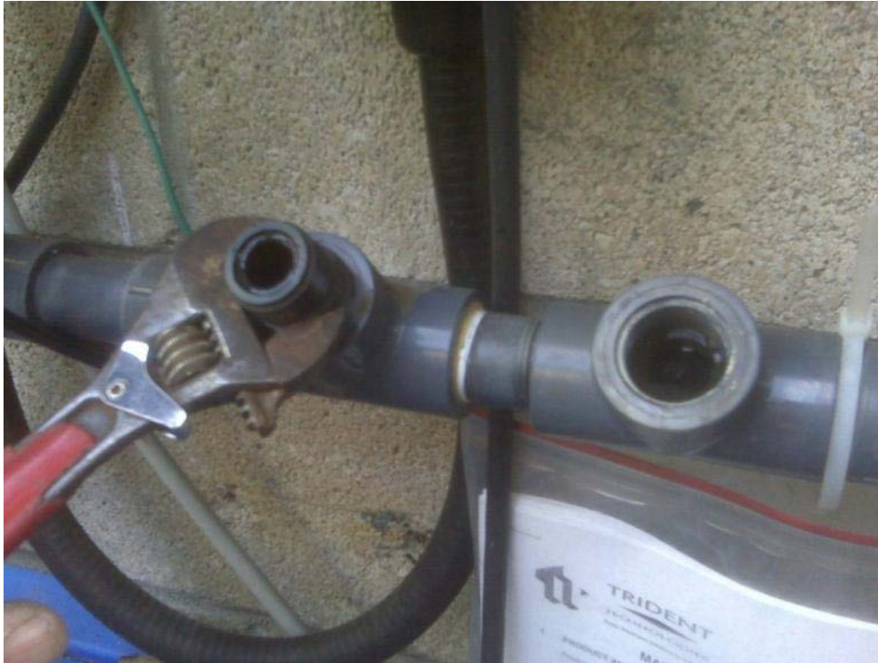
Remove old compression fitting
